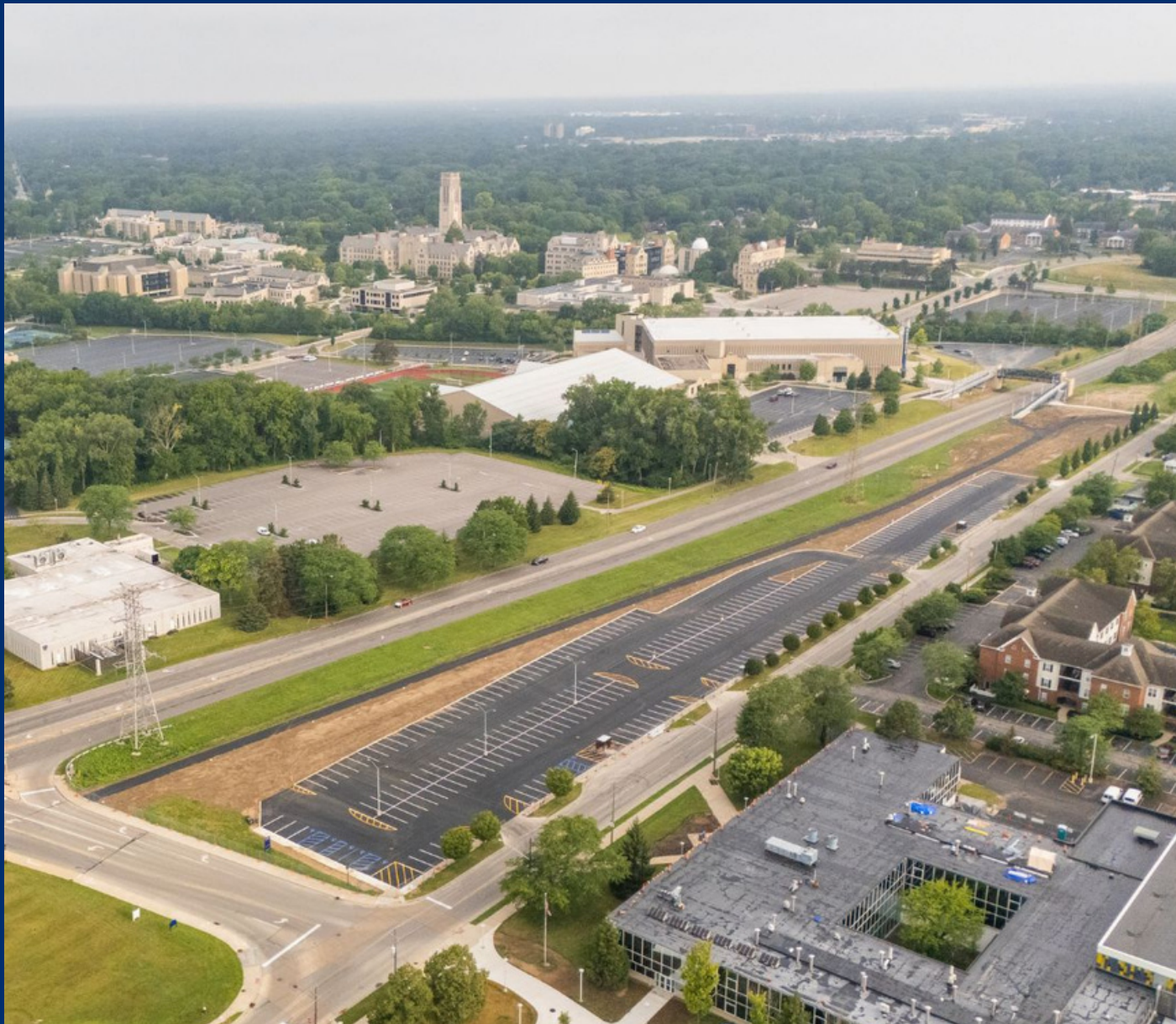
AERIAL VIEW OF AREAS 2, 3, 4, 18, AND 19 ON MAIN CAMPUS.
